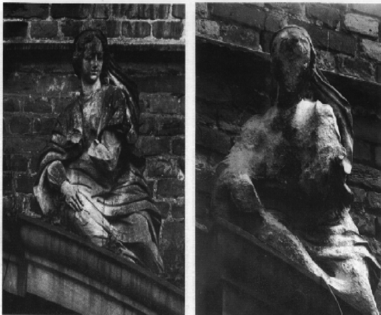
FIGURE 2.6 An example of acid precipitation damage to an outdoor statue. The statue, made of porous sandstone, was created in 1702 as part of the gable of the entrance of the Castle at Herlen, near Rocklinghausen, Germany. The left photo, taken in 1908, shows some stains and the loss of the left hand, but most of the face and right hand were intact after 206 years of exposure. The right photo, taken in 1969, shows the loss of most of the detail of the statue over 61 years [24]. (Reprinted with permission from the Westfälisches Amt für Denkmalpflege.)
